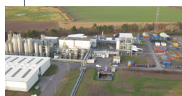
Wesseling, Germany ■ Production Plant
